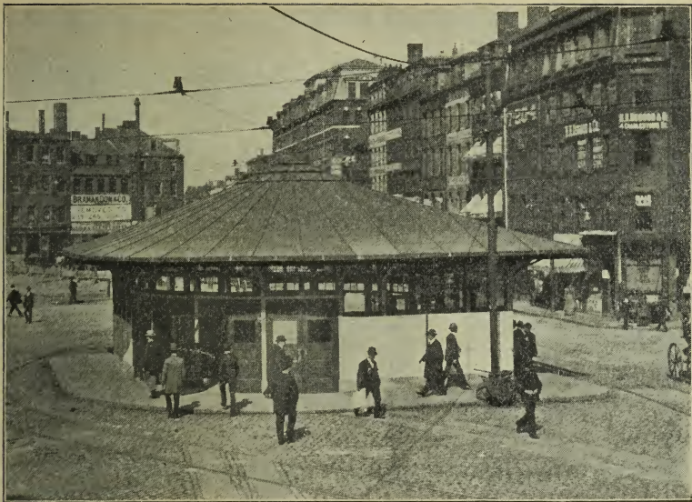
BUILDING OVER STAIRWAYS, HAYMARKET SQUARE.
